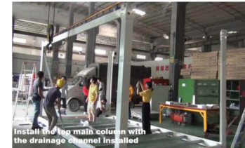
6.Install the top steel beam
