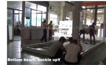
5.Install the column and the bottom tube
