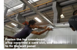
9.Install the top square pass
