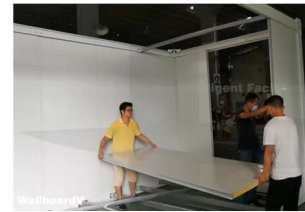
7.Install wall panels
